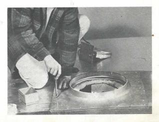
5. **ELECTRICAL CONNECTION** — Check the control mounting bracket to make sure it clears the top of the open damper blades by a minimum 1/8 inch. If the control bracket is in contact with the damper blade, a spacer will be required between the grille and ceiling as outlined in paragraph 3.
